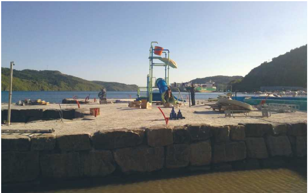
Ill. 1: The outdoor waterworld, "Sørlandsbadet". Construction site. (Photo: Sarah Holst Kjær)
