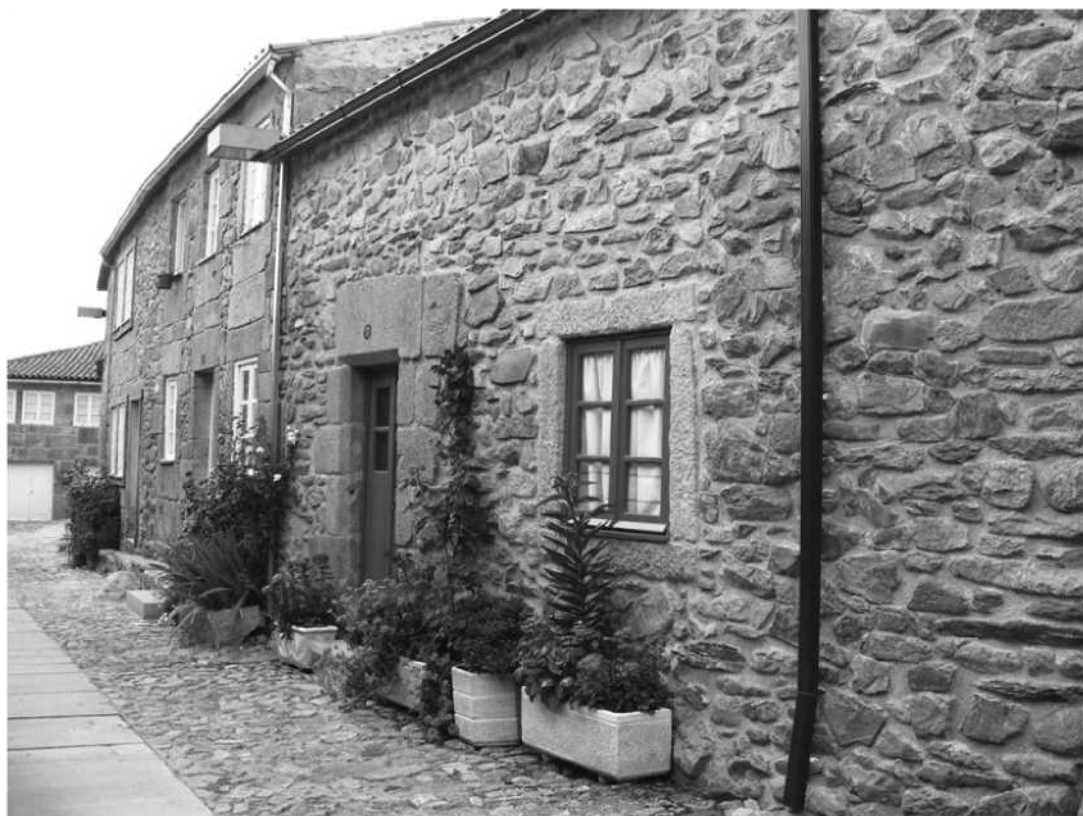
Ill. 1: Visible stonework and gutter pipes in the facades of houses in Castelo Rodrigo. (Photo: Luís Silva, 2009)
