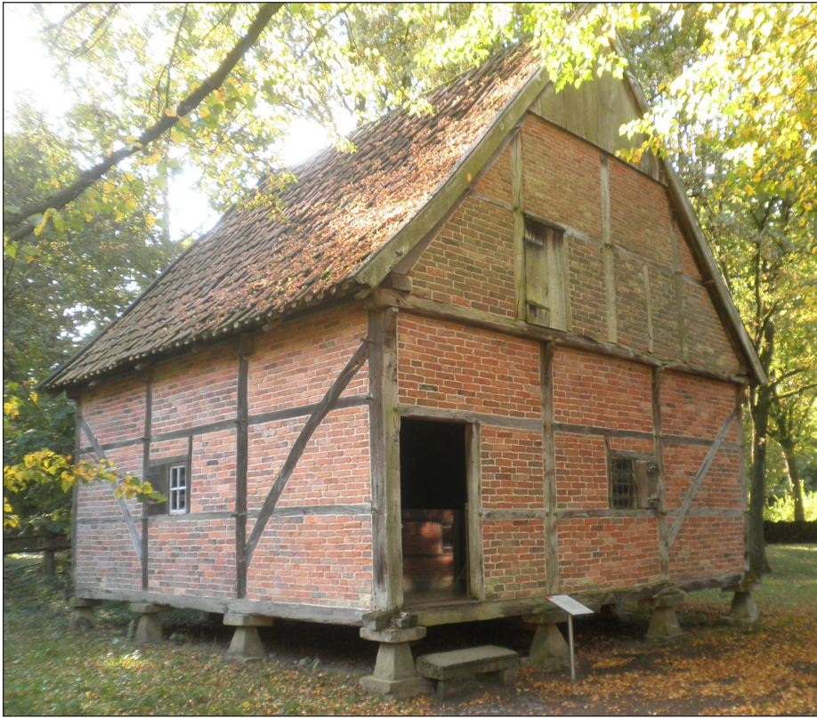
Figure 3: Structural protection against food competitors: On anti-mice pillars hovering granary built about 1820 in Lasbeck (County of Coesfeld), shown in the open-air museum in Detmold. (Photo: Michael Schimek)
