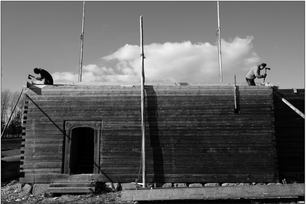
Figure 1: The reconstruction of the medieval timber church of Södra Råda, by using traditional methods and hand tools, primarily aims at a deeper understanding of the original church and its medieval context. (Photo: Gunnar Almevik, 2019)
