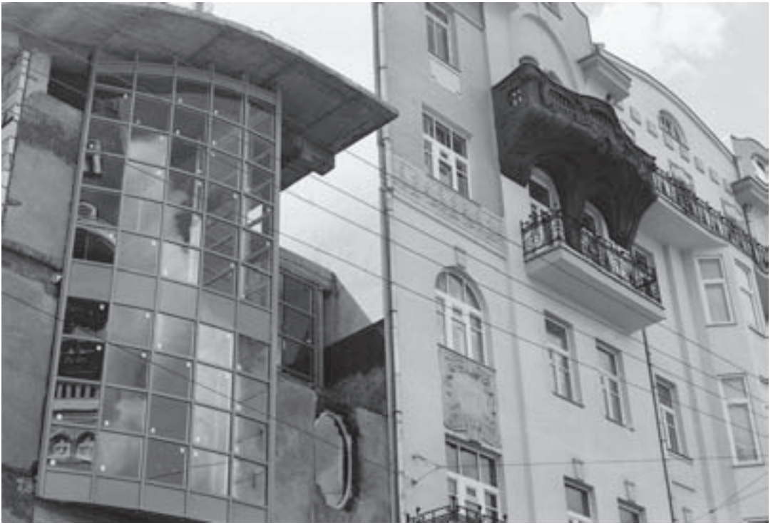
Renovation of art-nouveau tenements next to postmodern office constructions. Photo: Cordula Gdaniec 1996.
